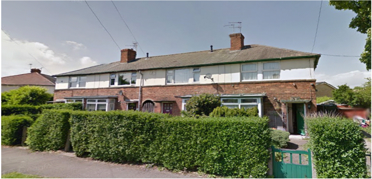
Figure 7 – Showing a Dennis Wilde Property on Burlington Avenue
