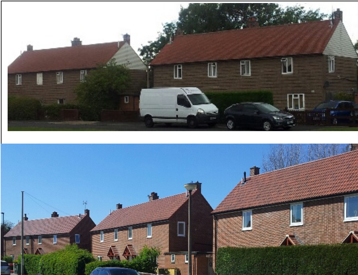
Figure 11 – Airey houses in Derwentthorpe as built (top) and post 2014 conversion (bottom)
